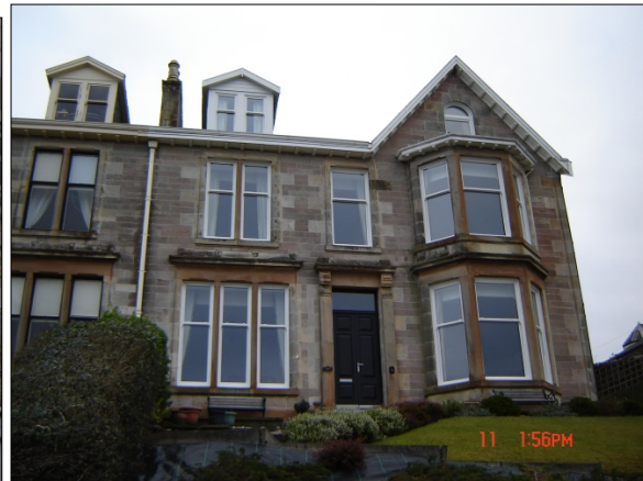
uPVC sliding sash Windows @ Crichton Rd
