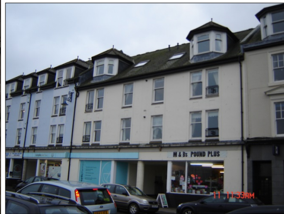
Timber double swing windows @ Victoria Road
