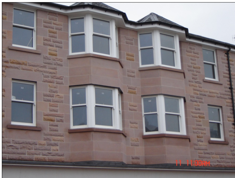
New timber sash and case windows @ Guildford Square
