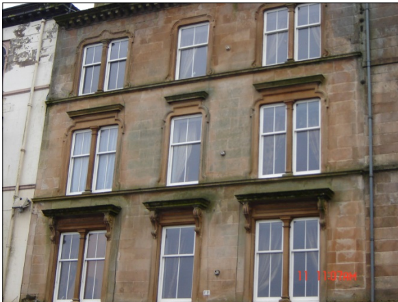
uPVC sliding sash @ Albert Place
