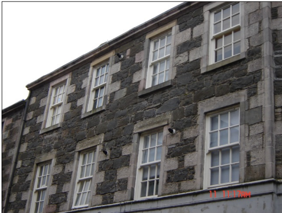
Timber swing windows @ Montague St
